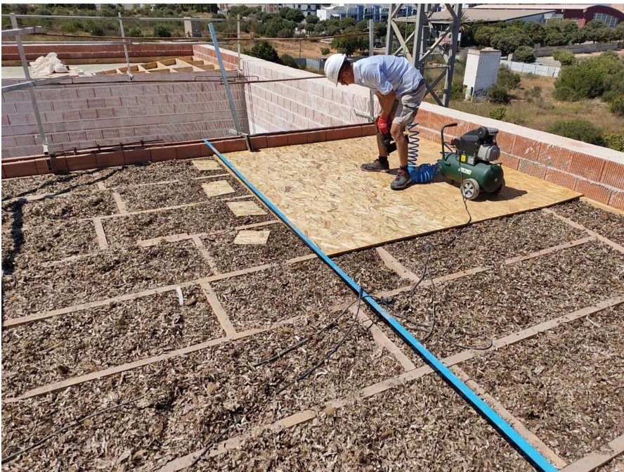
Adapting an ancient tradition of using posidonia as an insulation material, the scheme uses local seaweed on its roof Credit:Estudi 08014
