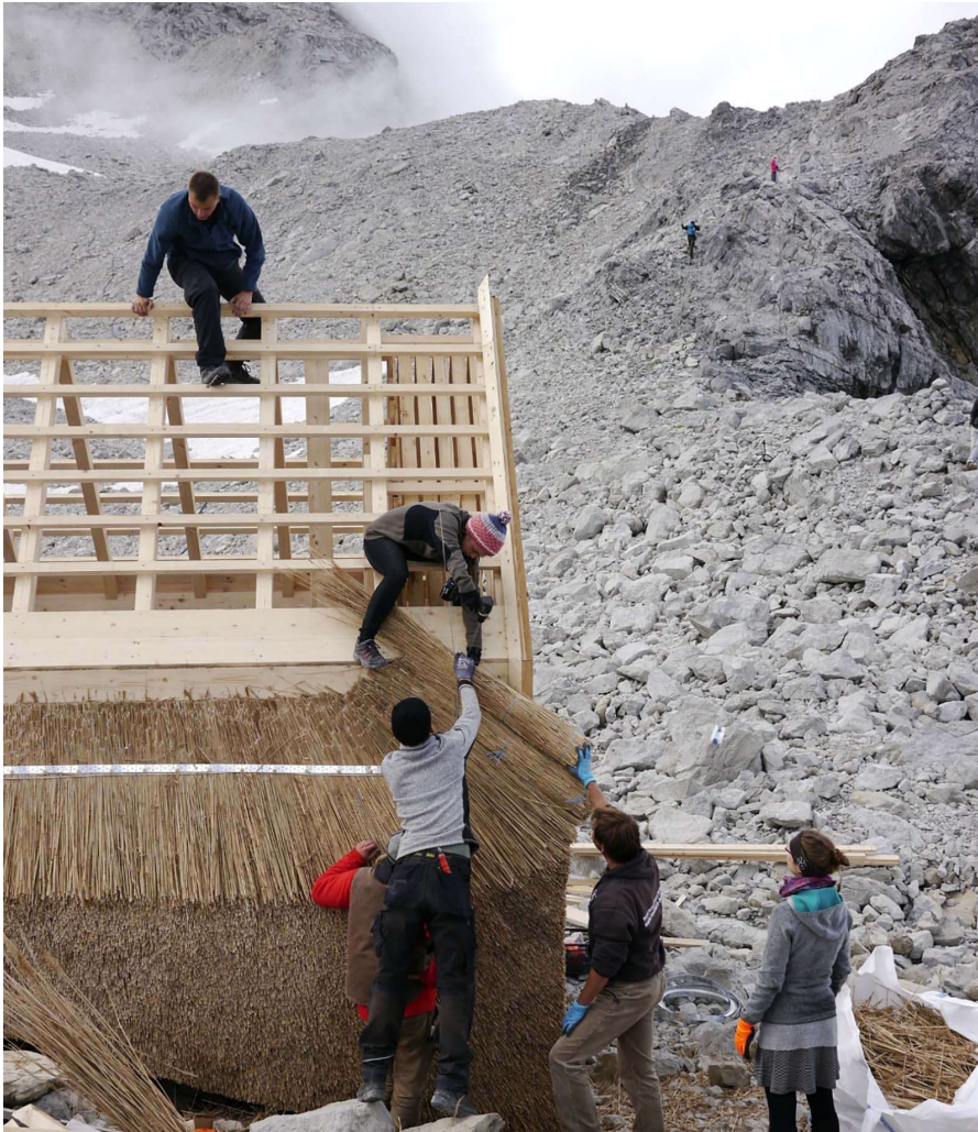
Reed is used to create a thatched outer skin for the University of Stuttgart's Alpine hut Credit:IBBTE / University of Stuttgart
