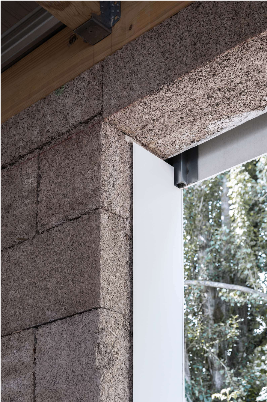
Hempcrete, as seen at a recent French sports centre by Lemoal Lemoal, is often presented as a viable alternative to concrete Credit:BCDF
