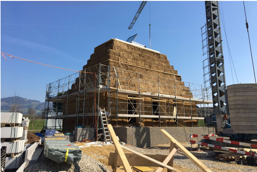
Atelier Werner Schmid's office building uses straw as a primary material Credit: © Atelier Schmidt
