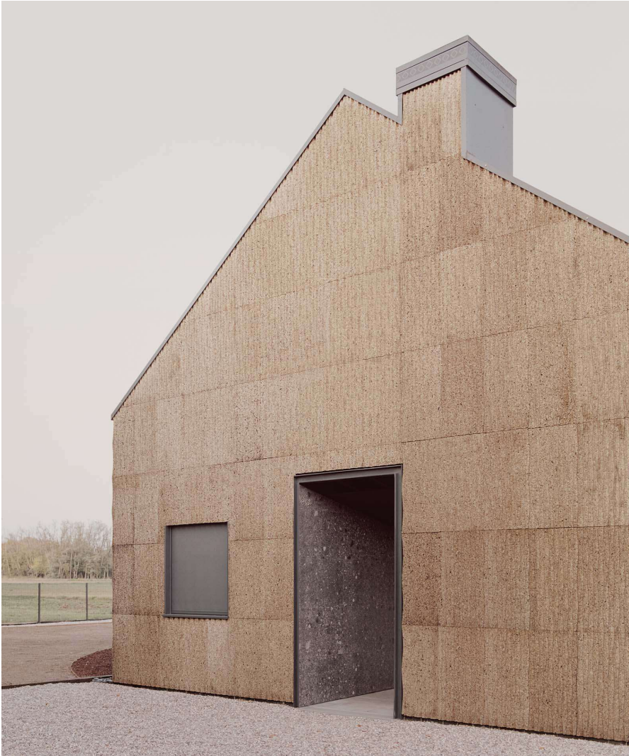
The House of Wood, Straw and Cork by LCA Architetti in Magnago, Italy, tackles three plant-based materials in one project, taking advantage of the different properties of each. Timber performs well as a load-bearing material, straw is suitable for insulation, and cork can readily be used as cladding Credit:Simone Bossi
