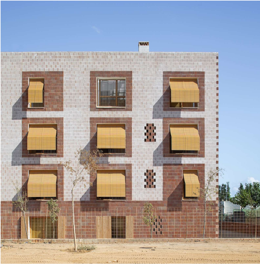
Seaweed is abundant in island locations such as Ibiza, where Estudi 08014 designed 24 public housing units in 2022, with the support of the Instituto Balear de la Vivienda (IBAVI) Credit:Pol Viladoms
