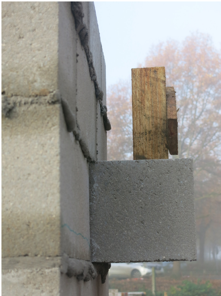
[Moke up blockwork with backflow joint / sculpture support]
