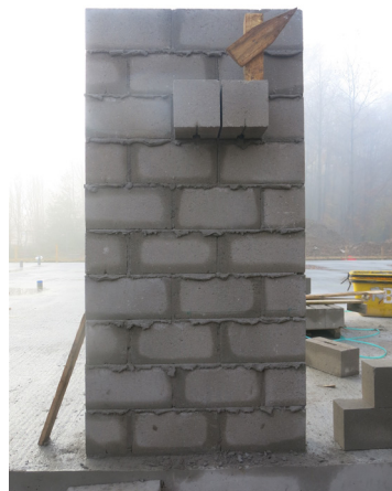
[11_Make up at the building site]
